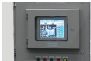
Monitor and alarm System
